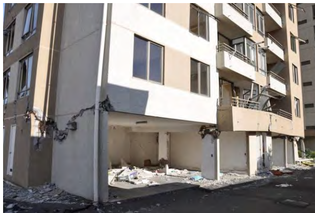
Figure 3.5-1 Coupled walls in upper stories do not continue to lower story (Plaza del Rio Building, Concepcion, Chile)
