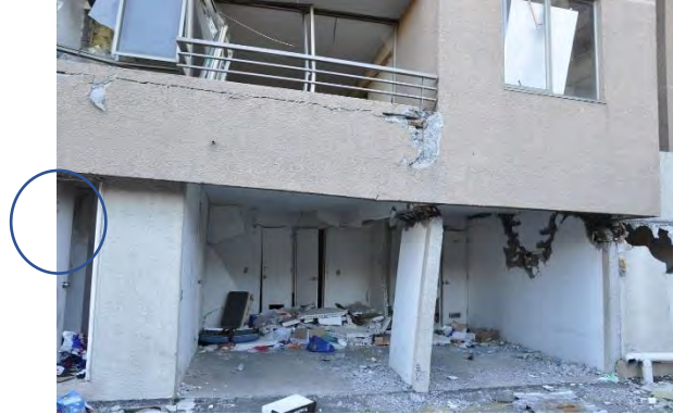
Figure 3.5-2 A change in the wall section from the upper to lower story (circled) results in a loss of wall area and localization of flexural yielding (Plaza del Rio Building, Concepcion, Chile)
