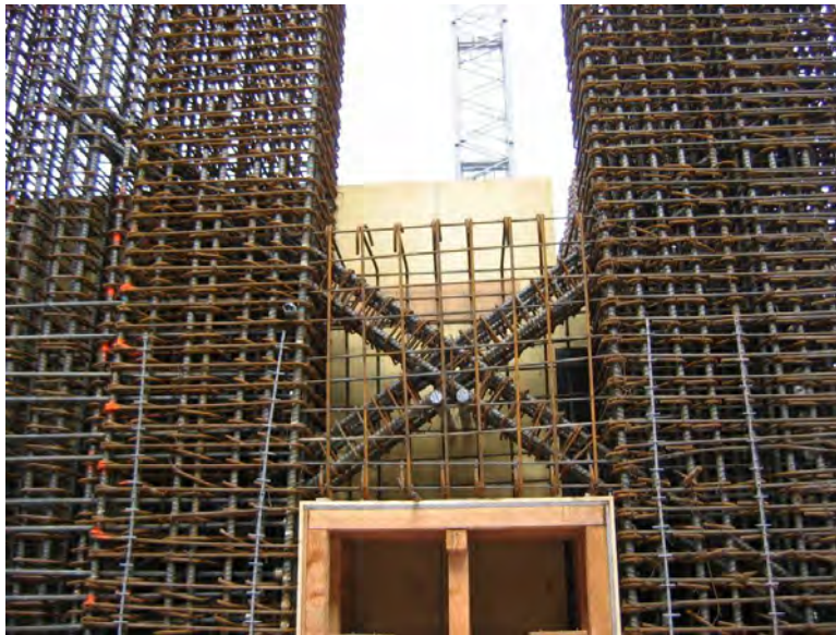
Figure 2.1-8 A diagonally reinforced coupling beam (Source: http://nees.seas.ucla.edu/pankow )
