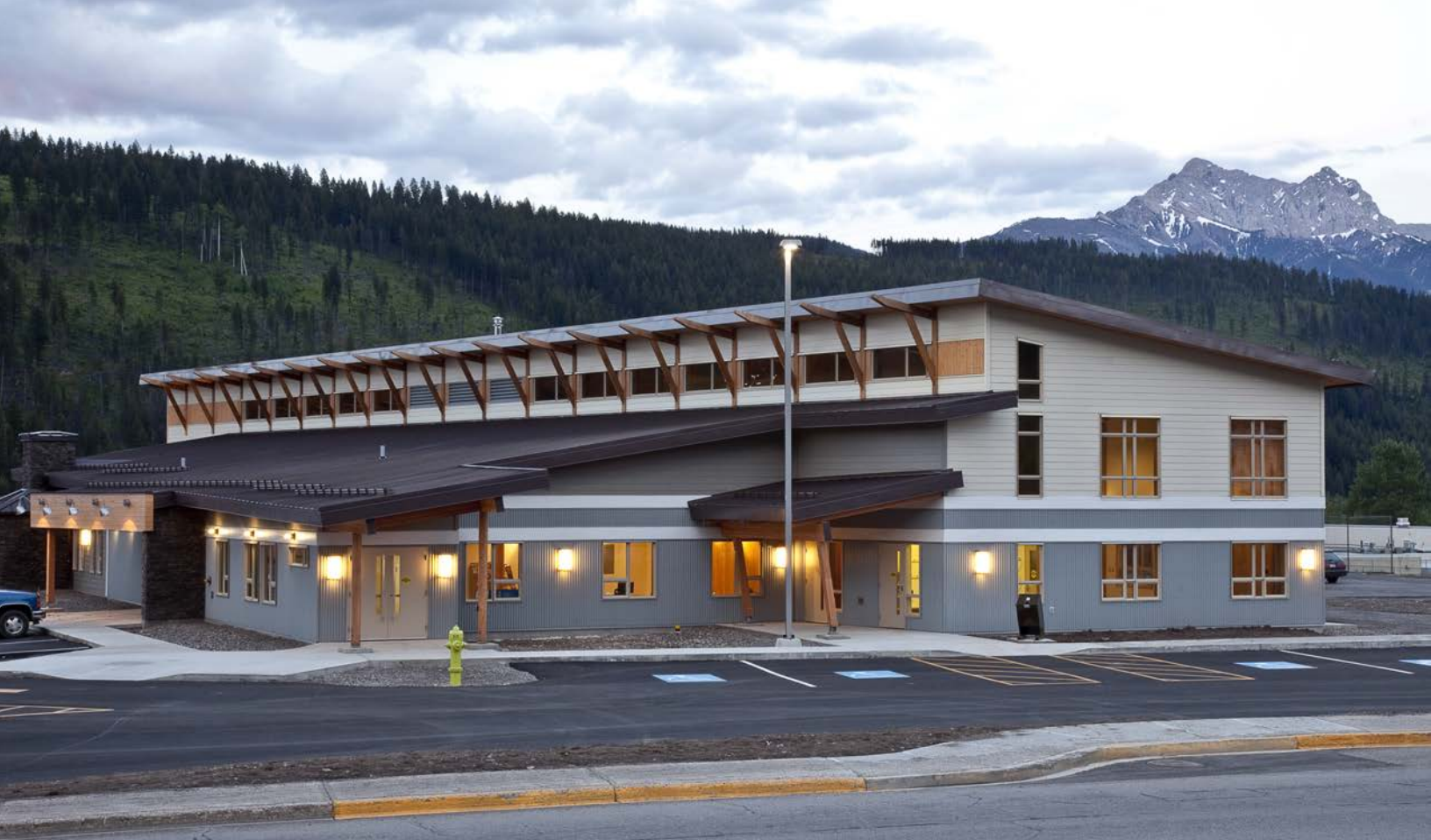
Elkford Community Centre Photo Credit: Douglas Sollows Architect Inc.
