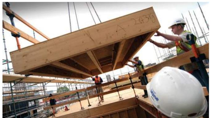
B) LANDING OF A PREFABRICATED FLOOR CASSETTE
